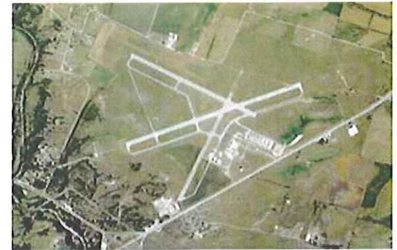
Temple Airport-hangar completed
