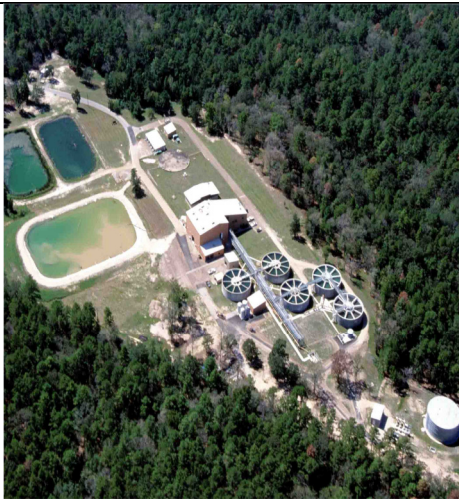
Proj Mgr: Trinity River Authority Huntsville Water Treatment Plant Expansion
