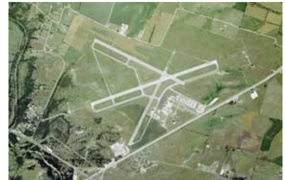
Temple Airport-hangar completed
