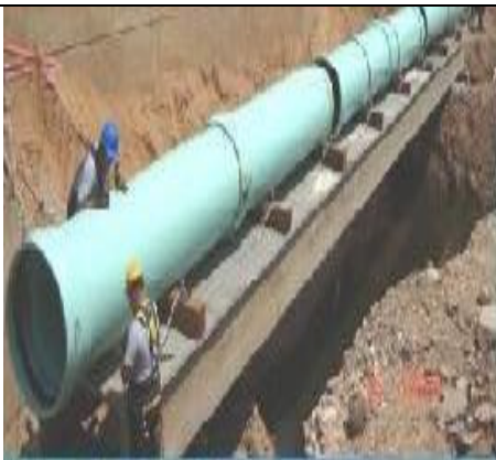
Prog Mgr: 36-inch Sewer Line
